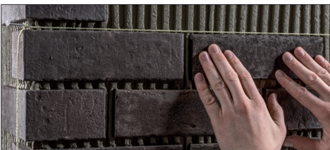
Placement of the surface clinker brick slips using a line aid. The clinker brick slips are pressed into the adhesive bed.
